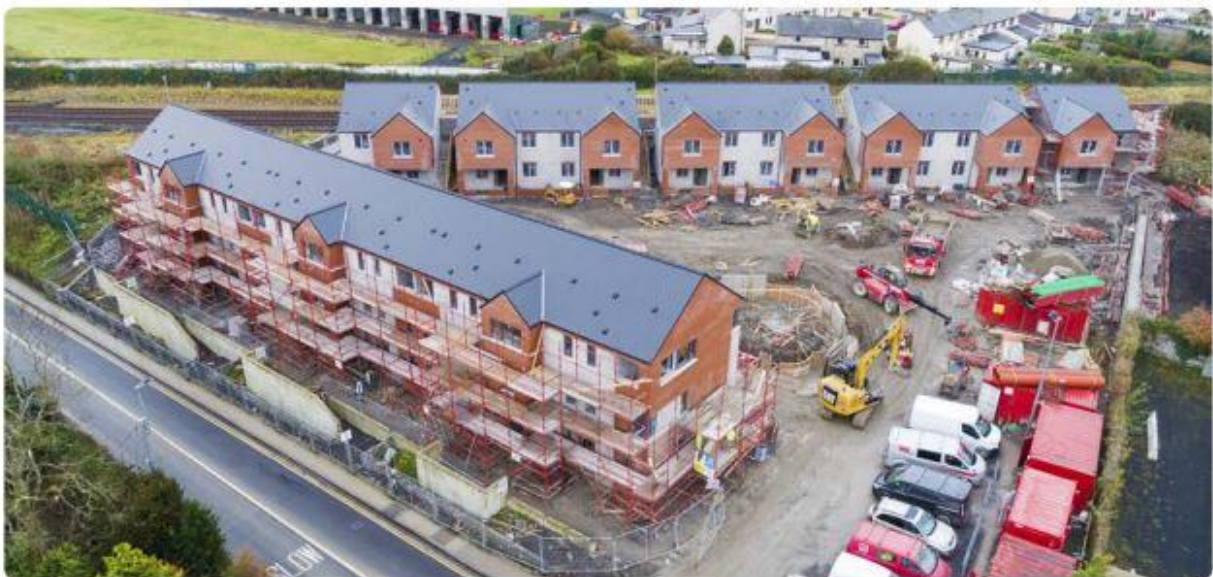
Knappagh Beg Court, Sligo Town – SCC project of 28 properties completed.
